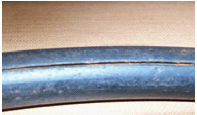
Failed pipe seam not due to freezing
