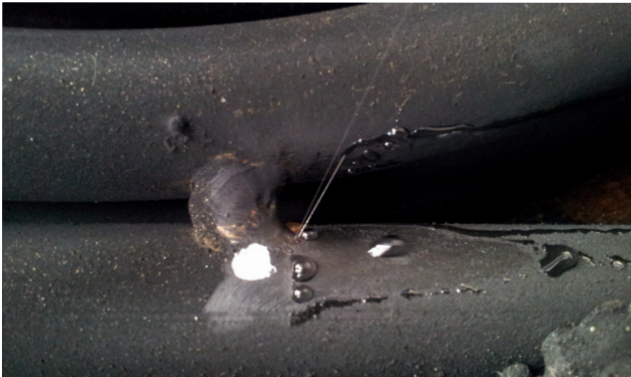
Failed weld, failed material, or pin hole not due to freezing
