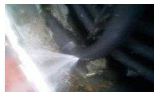
Blow out from pipe weakened by freezing
