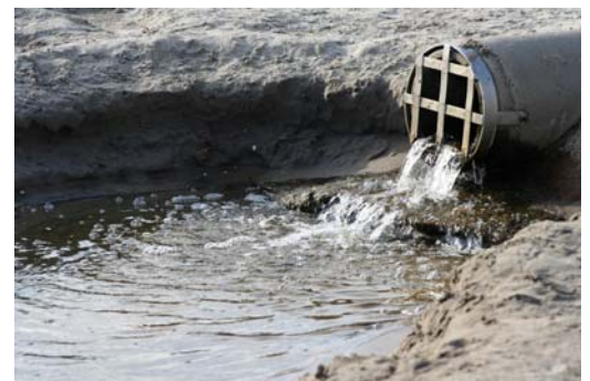
Thaw and clear ice from drains and culverts
