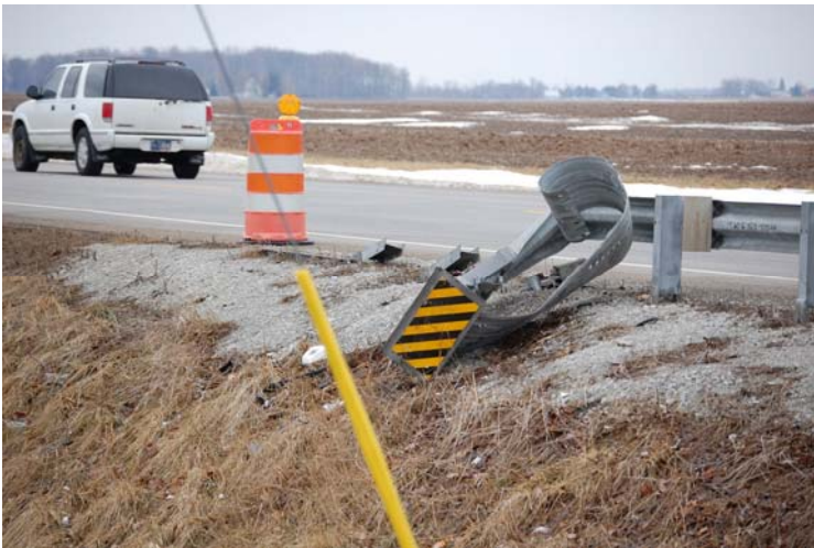
Guard rail stump removal – hot water pressure washer cuts through ice and thaws area around stump
