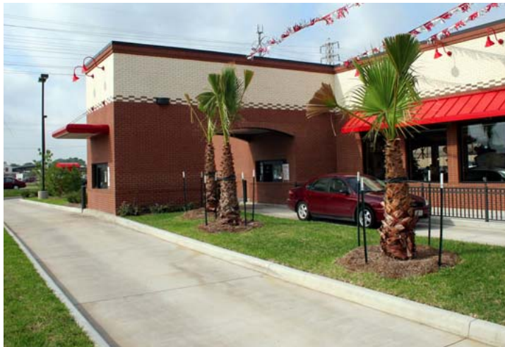
Store front & dumpster area cleaning & washing
