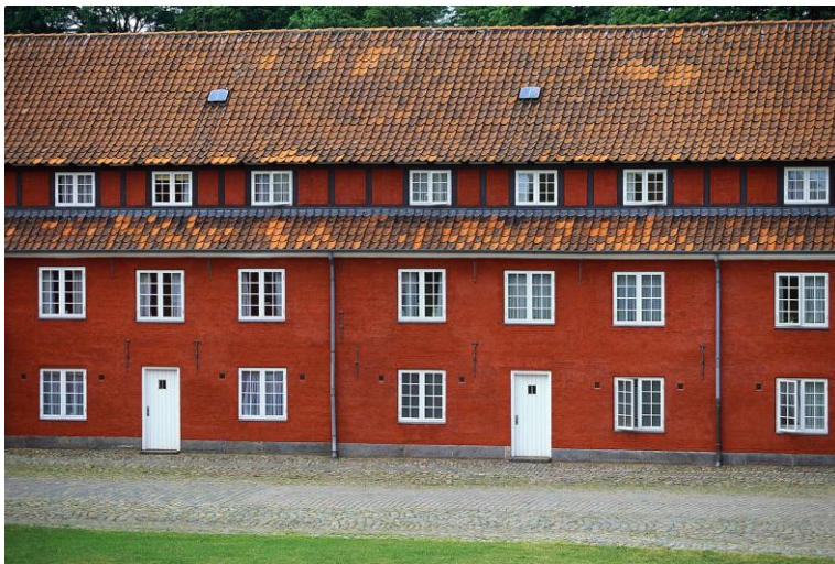
Two gun building, roof and concrete cleaning & washing
