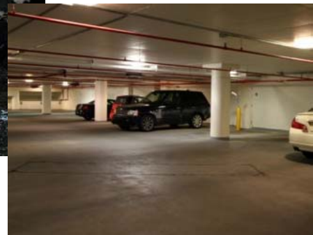
Parking garage cleaning
