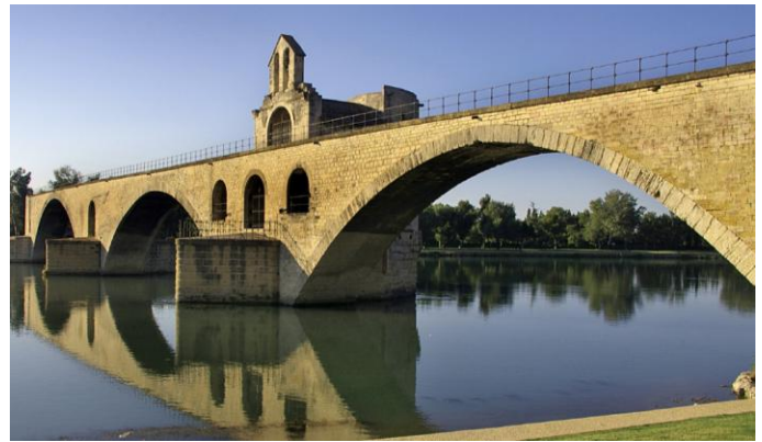
Bridge cleaning & washing
