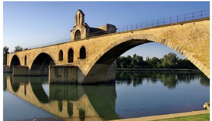
Bridge cleaning & washing
