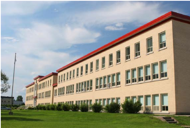
Multi-story commercial building cleaning & washing
