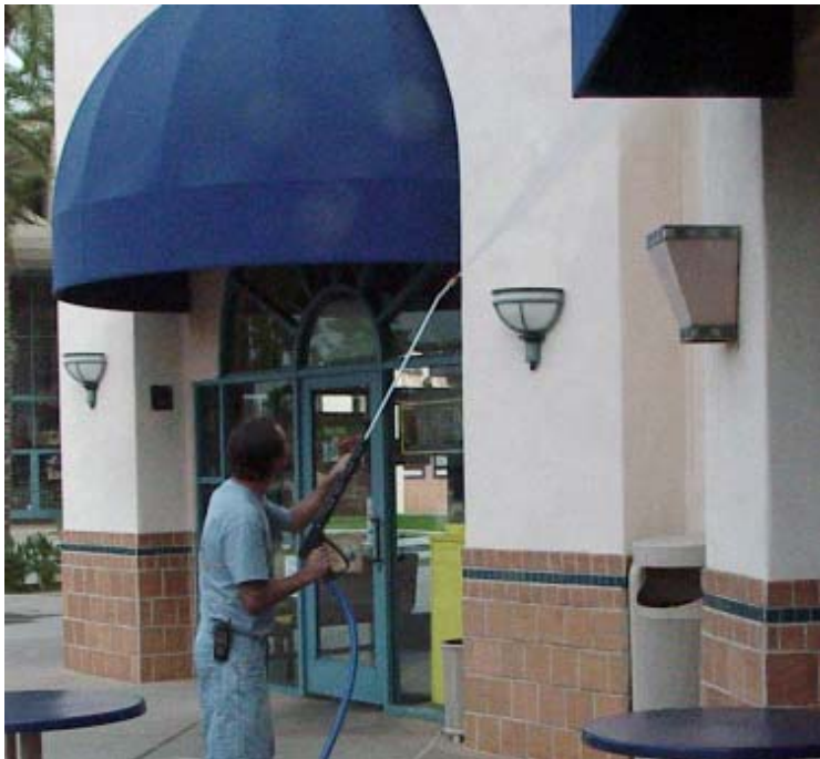
Building & shopping center cleaning & washing
